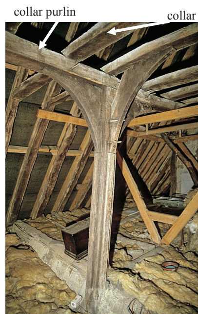
Fig 3: Crownpost on centre truss of open hall at Railway Terraces, Wenham, Suffolk
