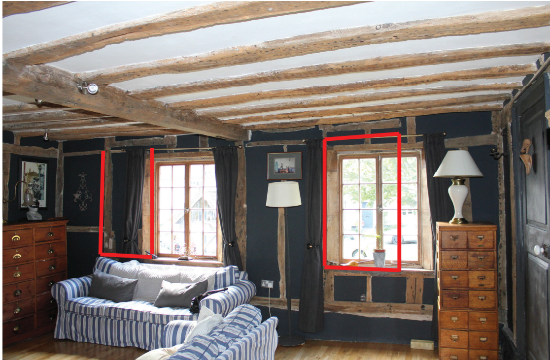
Fig 6: South wall on ground floor of service end with original windows highlighted
