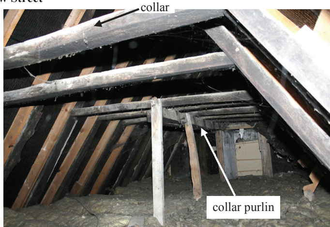
Fig 4: Heavily smoke blackened roof over the hall of 23 Low Street looking south. The crownpost has been removed and the collar purlin truncated.
