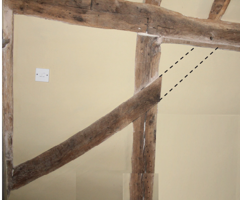
Fig 8: Convex or drooping brace in 24 Low Street
