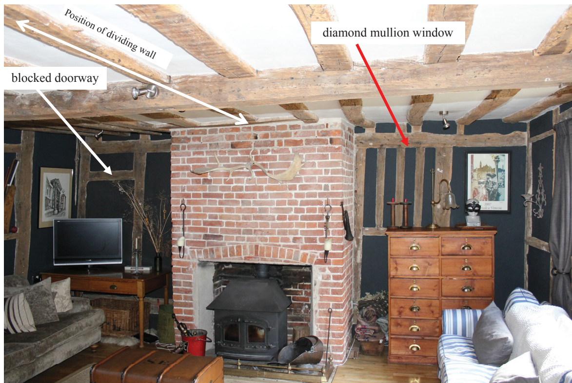
Fig 5: South wall of service bay. the partition between the two rooms has been removed and the chimney stack inserted in the 18 th or 19 th century
